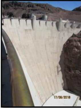
dam for a two lane highway from Seattle, WA to Miami, FL or a 4ft. wide sidewalk around the earth at the equator. At its base it is as thick as two football fields measured end to end. It is 1244 feet across, 45 feet thick at the top, and is 726 feet tall. That's almost 200 feet taller than the Washington Monument in Washington, D.C. Today, the Hoover Dam is the second highest dam in the country and the 18th highest in the world. It generates more than four billion kilowatt-hours a year, that's
